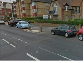
when placed either side of a junction the give way line can be brought forward to improve visibility for emerging vehicles.
