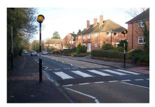
Where pedestrians are having difficulty crossing a road, a new zebra crossing may be a suitable solution to deal with this issue. They consist of dropped kerbs, tactile paving, belisha beacons on posts and sometimes high friction surfacing on the approaches to help vehicles stop quickly.
