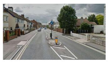
Where pedestrians are having difficulties crossing the road, an alternative to a formal pedestrian crossing is a refuge island. This allows pedestrians to cross the road in two halves and is particularly useful on busier roads where getting a gap in traffic in both directions at the same time is difficult and where a zebra or puffin crossing is not warranted.
